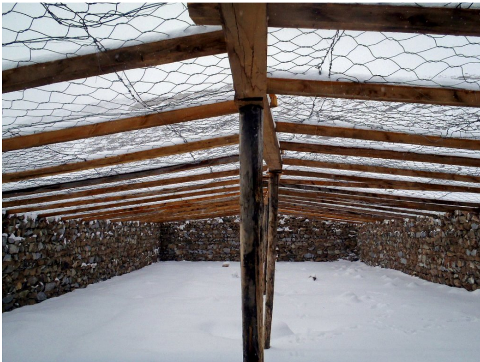
Figure 2. Communal predator-proof corral in Eshkili , Little Pamir. Top – External view of the walls of the corral. Bottom – Inside view of the corral showing the wide mesh size of the wire-mesh on the roof to avoid snow accumulation and roof collapse, November 2018.
