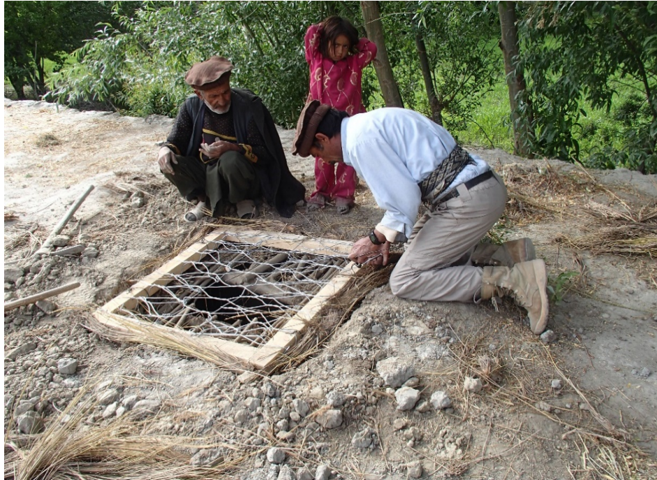
Figure 4. WCS snow leopard team member, Aziz Beg, fixes a one square-meter wire-meshed wood frame over a ventilation hole of a household corral in Kret Village, Wakhan National Park. Snow leopards have been reported to break into corrals through such ventilation holes, when not protected, July 2015.
