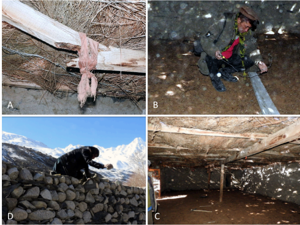
Figure 5. Maintenance work carried out on the communal corral of Kuzget Village on 16 November 2018. A&C – Broken timber before and after change. B&D – WCS team changes broken timbers in Kuzget corral. Note – Because the beneficiaries have added dry vegetation on the wire-mesh roof, which has not been designed to withstand the weight of snow, winter snow weights heavily on the roof structure, explaining the premature breakage of timbers.
