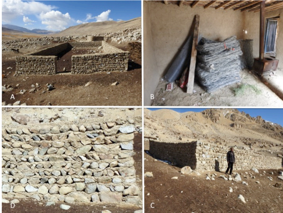
Figure 3. Communal predator-proof corral in Tila Bai , Big Pamir. A&C – External view of the walls of the corral. B – Wire mesh for the roof and door stored for winter and to be installed in summer 2019. D – Detail of the masonry stone and clay walls, 2 October 2018.
